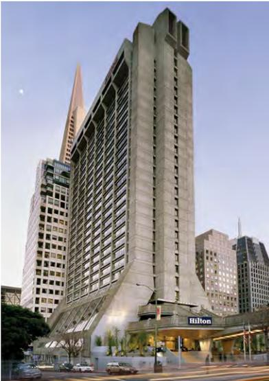
This was a fast-track renovation of 550-guestroom hospitality project with four floors of public spaces that entailed new design-build MEP systems, modifications to the porte-cochere and exterior waterproofing repairs.
