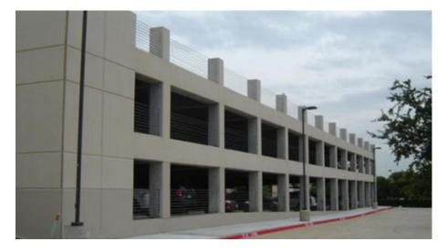
Marx|Okubo led a repair design and reconstruction effort on this recently constructed garage that had begun showing signs of unusual and excessive slab heaving and unevenness. Our investigation efforts led to an effective solution that involved slab demolition, base material remediation and doweled reconstruction, tying the new elements into the existing structure.
